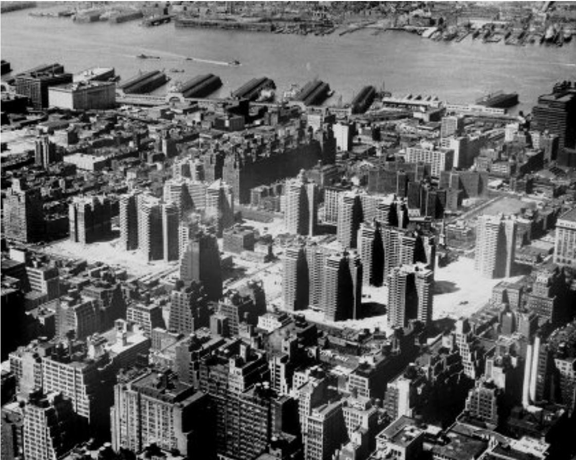
Penn South Construction Photo
